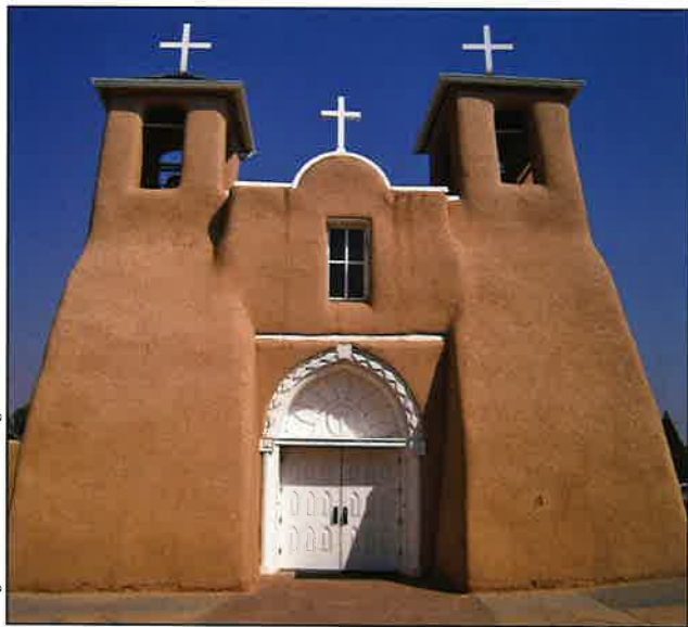
Catholic Spanish missions such as this one in Ranchos de Taos, New Mexico were constructed throughout the southwestern United States using local adobe building materials.
