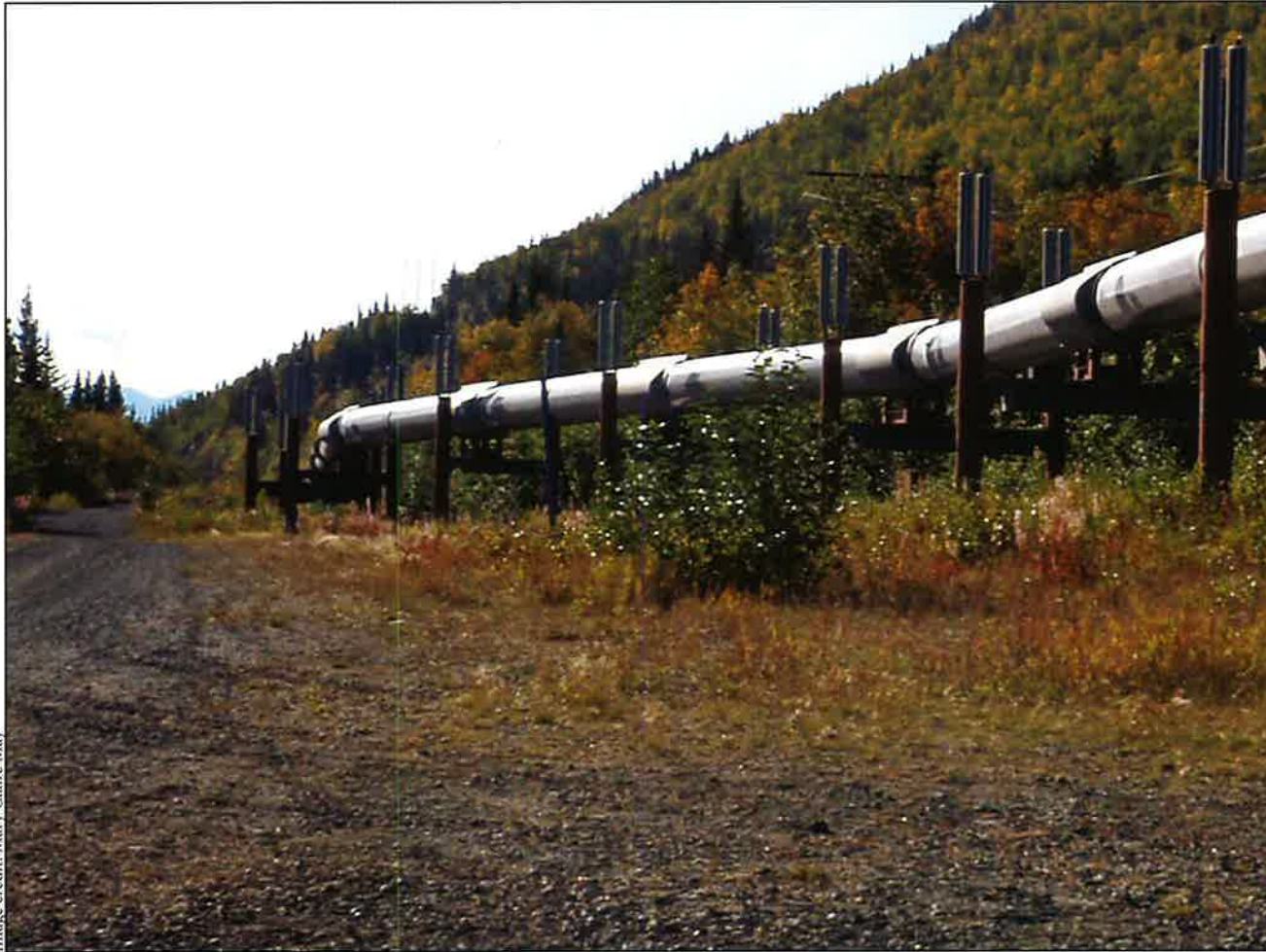
A segment of the 800-mile-long Trans-Alaska Pipeline System winds through the wilderness making connections between Prudhoe Bay and Valdez for the transport of oil.
